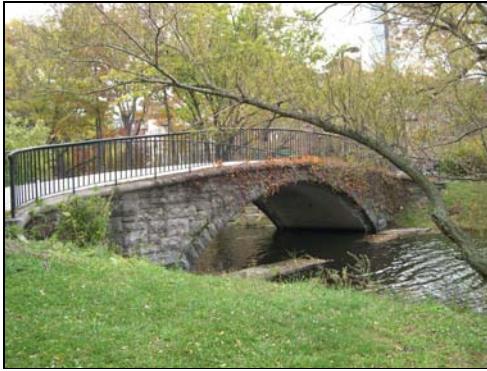
Figure 2.31 – 1930s granite bridge with new railing. (2007).
