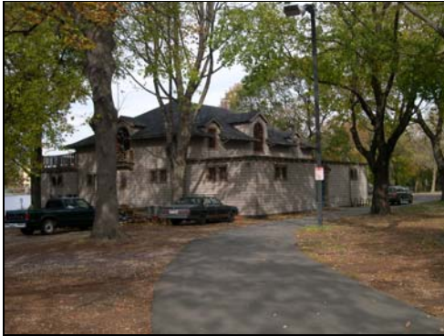
Figure 2.30 – Union Boat Club building looking northeast. (2007).
